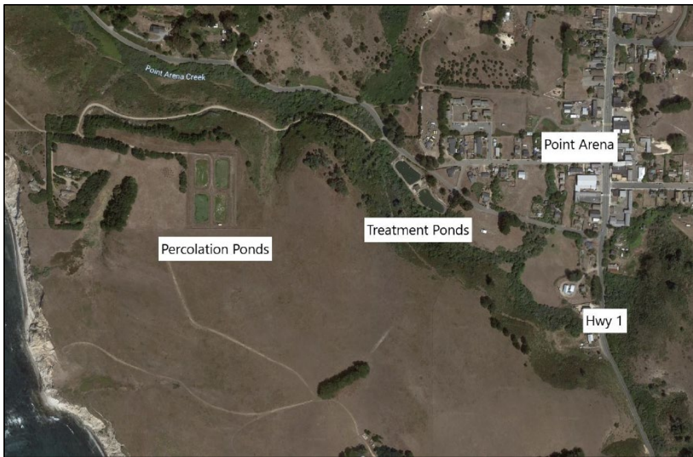
Figure 3-5: Point Arena WWTP Facilities
