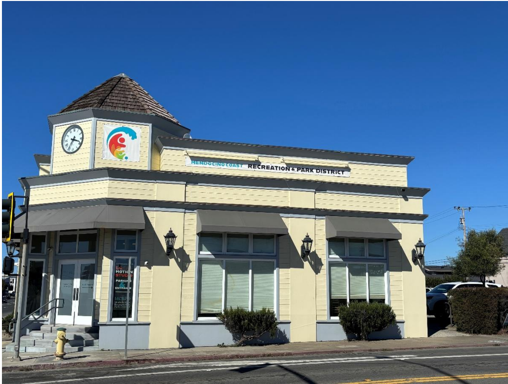
Figure 3-5: MCRPD Headquarters and Gymnastics Space
