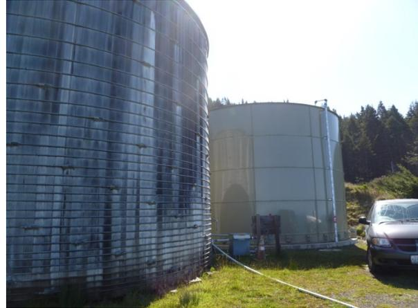
Additionally, the District has a 100,000 gallon Redwood Water Tank. The Redwood Water tank is in a state of degradation and is leaking. Staff has identified two solution alternatives: line the tank; or repair the floor of the tank. The District currently has no funding for completing either alternative and continues to monitor and temporarily patch the leaks as best it can.
